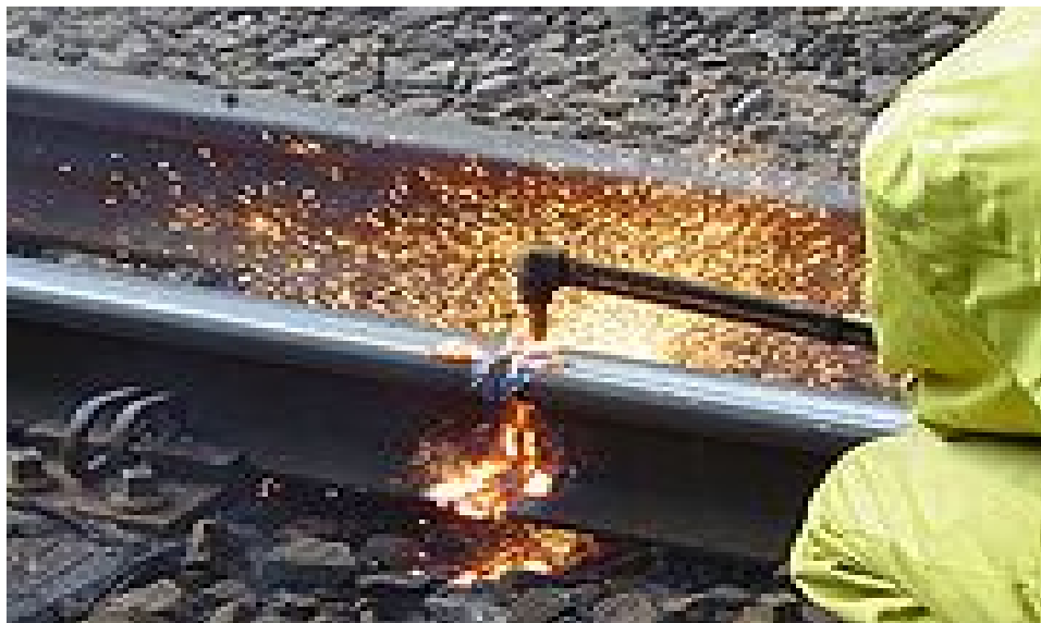
Fig 7 Manual Gas Cutting
