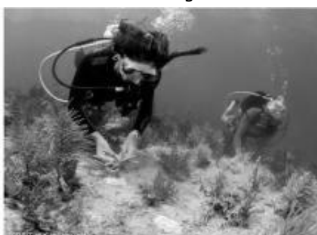
Repairing of the coral using cement and epoxy
