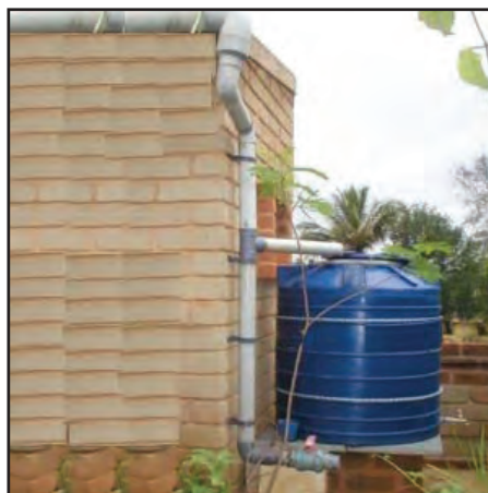
Rain water harvesting - a model
