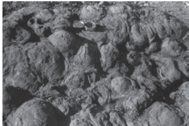
Fig.6.4 : Exfoliation (Flacking) and granular disintegration
