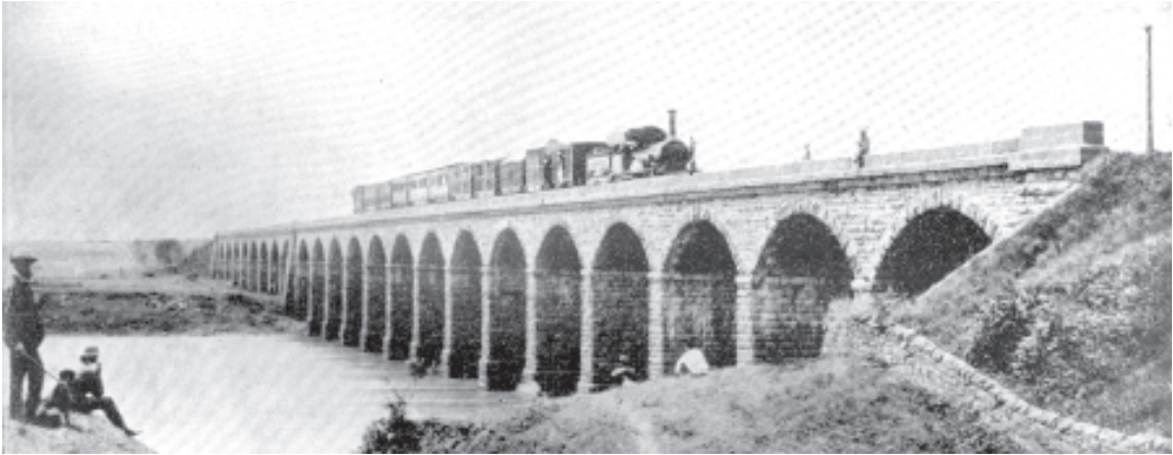
Fig. 1.4 First Railway Bridge linking Bombay with Thane, 1854
