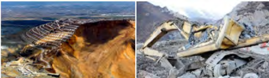
Fig. 6.6: Landslide hazards associated with mining
