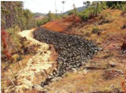
Fig.8.15: A buttress at the toe of a slope
