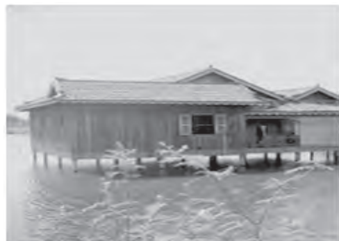
Fig.8.9: A house constructed in flood zone.
