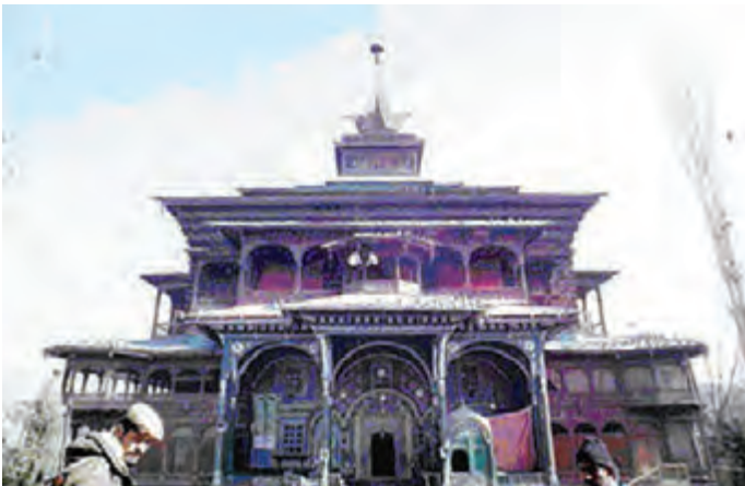
Fig. 6.11 The Shah Hamadan mosque in Srinagar, on the banks of the Jhelum, is often regarded as the “jewel in the crown” of all the existing mosques of Kashmir. Built in 1395, it is one of the best examples of Kashmiri wooden architecture. Notice the spire and the beautifully carved eaves. It is decorated with papier mache.
