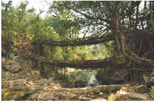
Fig 1.18 Root Bridge in Meghalaya
