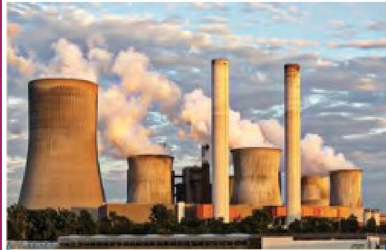
Thermal power station
